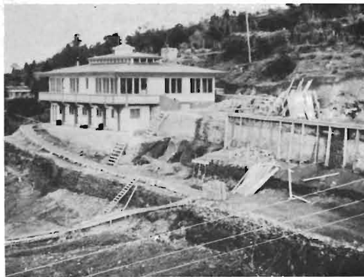
Sonada under construction
