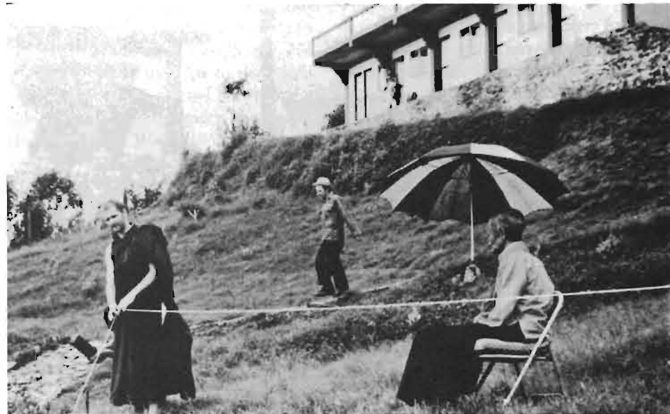
Supervising construction at Sonada, 1981
