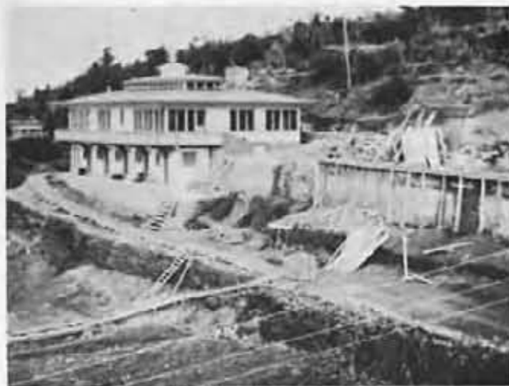
Sonada under construction
