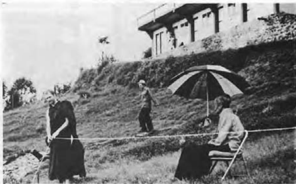
Supervising construction at Sonada, 1981
